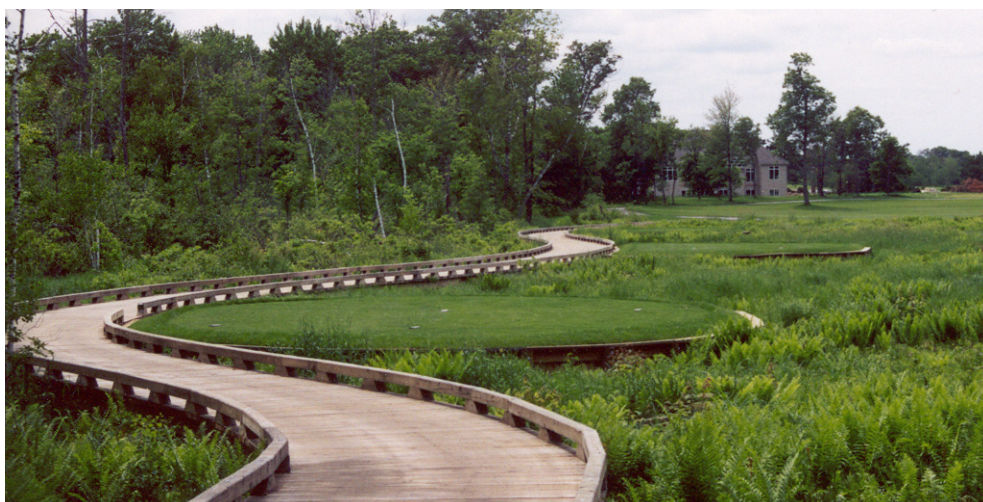
Wetlands like this one on No.17 at The Refuge in Oak Grove serve as stormwater detention areas and natural filters for stormwater runoff from surrounding roads and residential developments.
